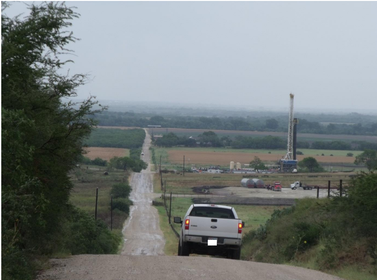
Figure 6: Drilling rig used in well excavation, Eagle Ford Shale, Texas
